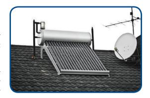
Most solar water heaters have three parts: a hot water storage tank, a solar collector that absorbs light from the sun, and a backup gas or electric heater that can heat the water in case of a cloudy day. Look at the picture of the solar water heater. It is designed to absorb as much light as possible and reflect as little light as possible.
