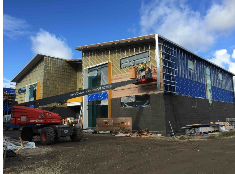
Classroom wing C
