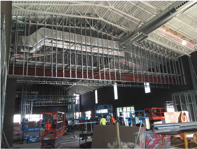
Interior view of Gym
