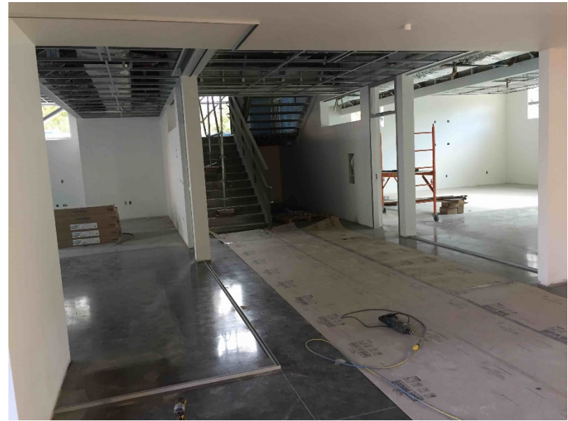
Interior Classroom wing C
